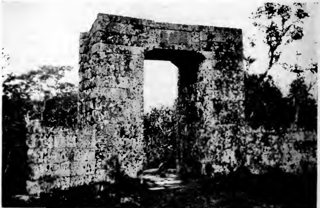
In the region of the coastal Loi of Hainan all villages and many estates have great gateways made of the lava-stone with which the district is overrun
